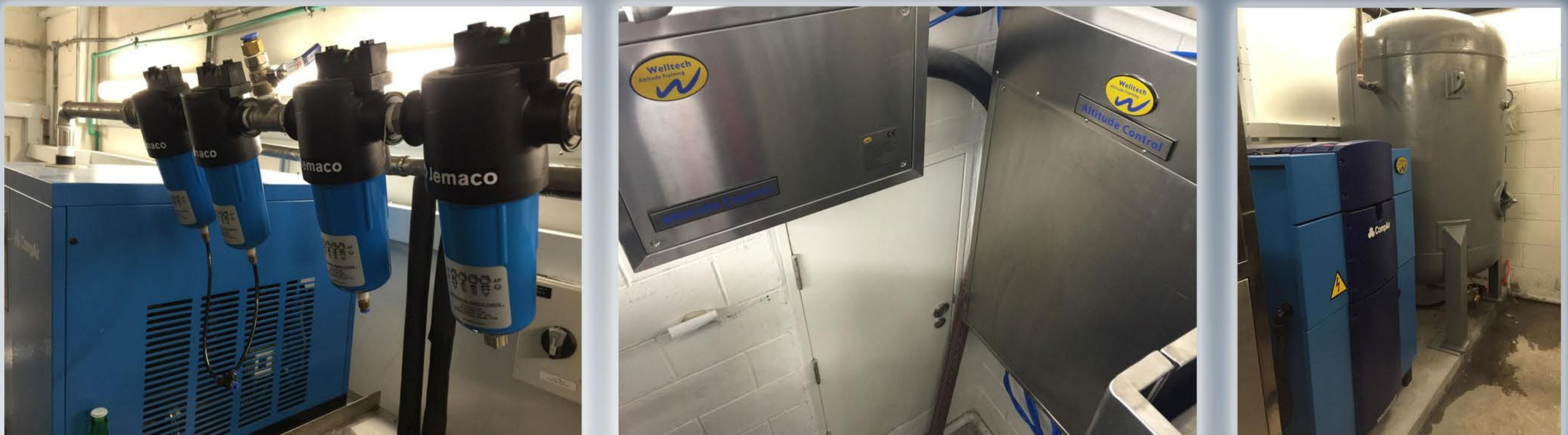
The no. of membrane, capacity of air compressor and dryer is depends on the room volume and its altitude control. The hypoxic system is custom design for different application. Consult Welltech for more detail .
